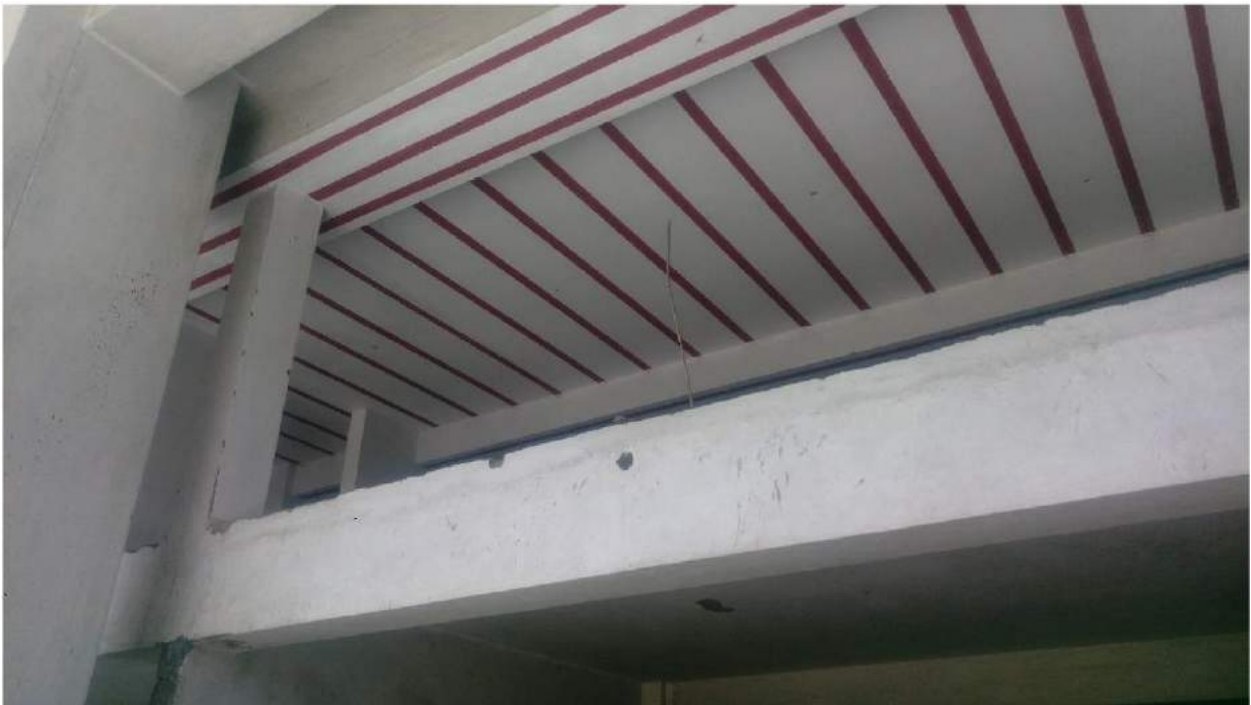
Undercoat painting and marking of PT strands
