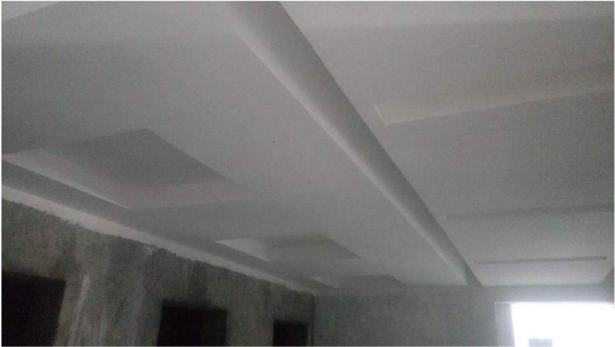
Sample of gypsum ceiling at the lift lobby
