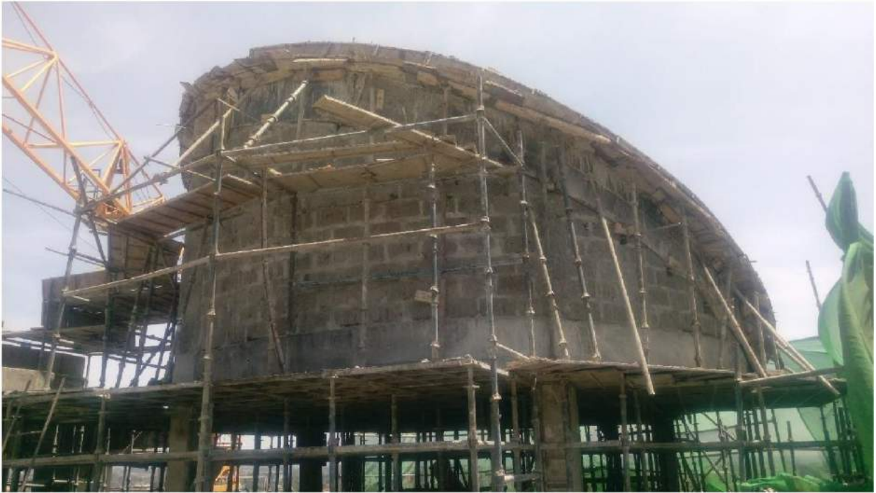
Works at the roof terrace
